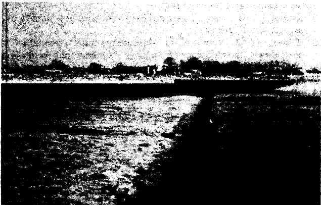
Figure 10 Free flow over a large flow-measuring structure
